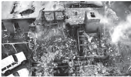
The Delta Upsilon fraternity at the University of Massachusetts at Amherst was destroyed by a fire started by an unattended candle. In addition, smoke alarms in the building had been covered by plastic and tape so that they would not be activated during parties.
